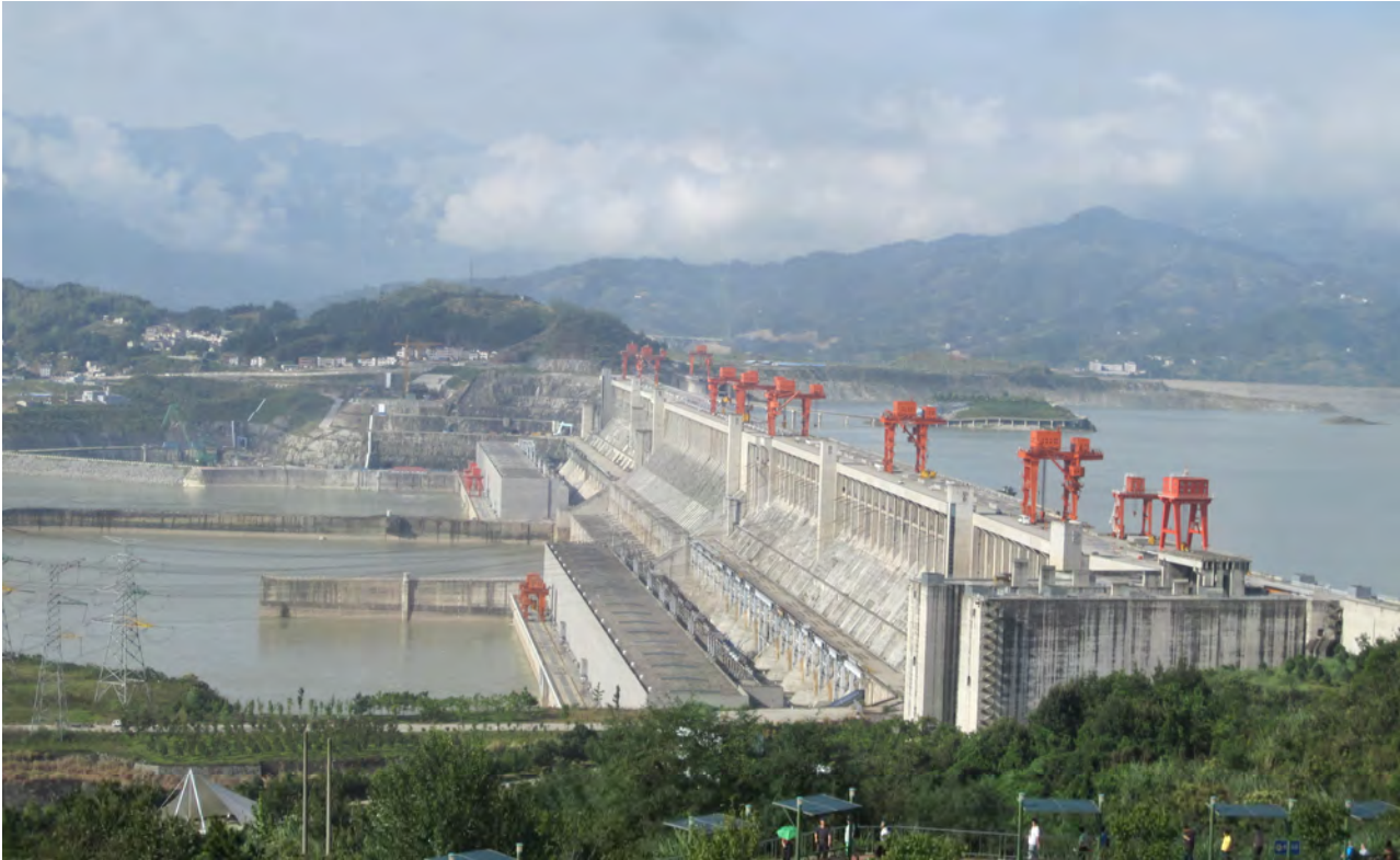
Figure 1-9. Most of the electricity worldwide is produced by three-phase synchronous generators. The above picture shows the Three-Gorges Dam hydropower plant, on the Yangtze River, in China. It contains thirty 700 MW three-phase synchronous generators, each weighing about 6 000 000 kg (about 6000 tons).
